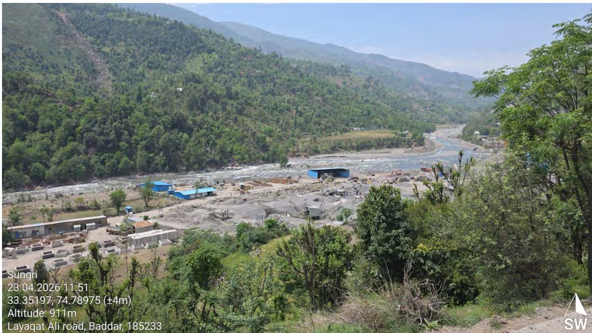
Pic-13: Construction Company Camp site.
