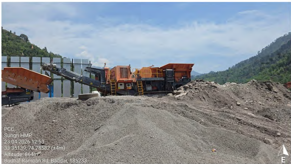
Pic-4: Mobile Stone Crusher
