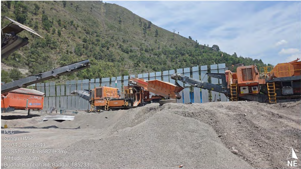
Pic-5: Mobile Stone Crusher
