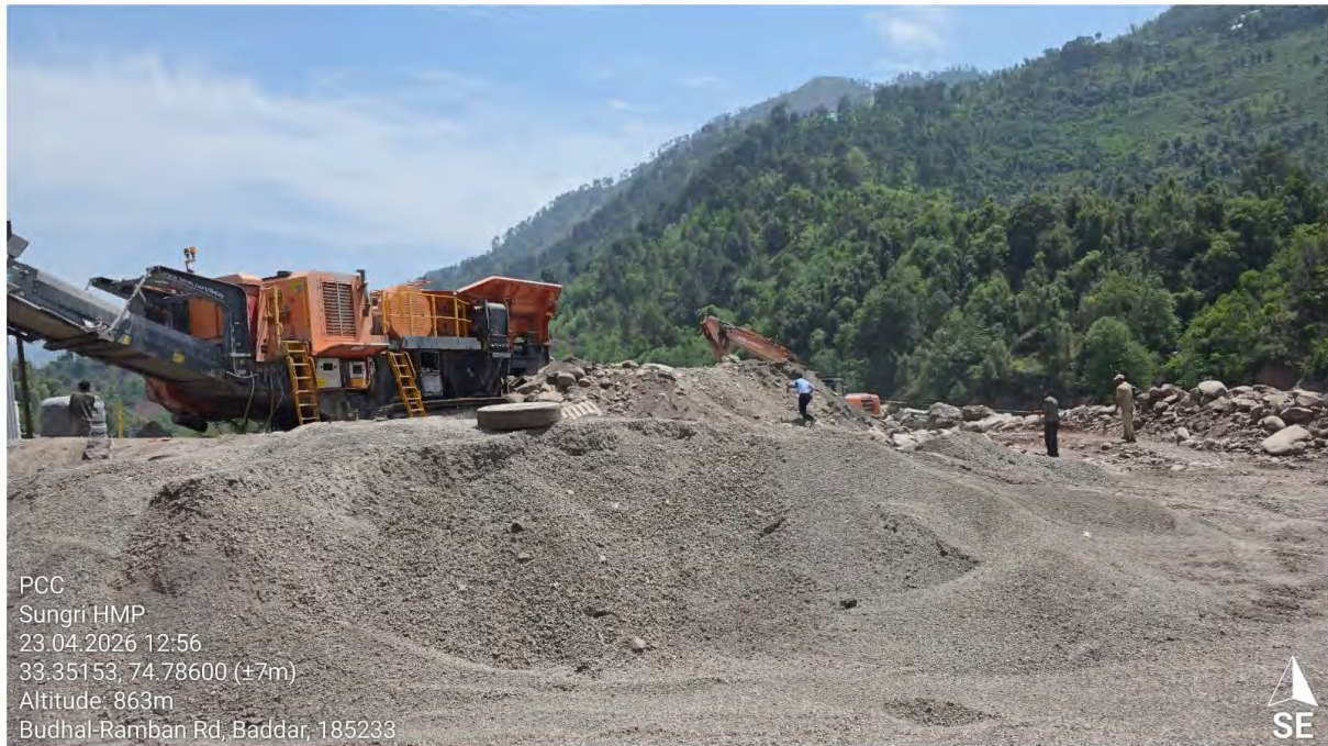
Pic-3: Mobile Stone Crusher
